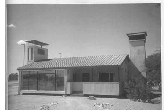
Figure 5-5. The Arizona test building with the evaporative cooling solar chimney (left) and a tower (right).
